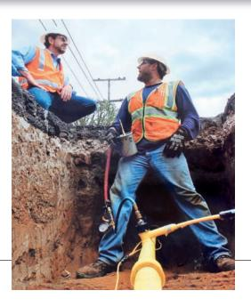
**Problem:** Insecure connections compromise the traceability of buried tracer wire and lead to expensive "dig-ins."
